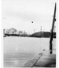
April 22, 1951 flood showing the Adams Company. Unpublished photo courtesy: Bob Reding
